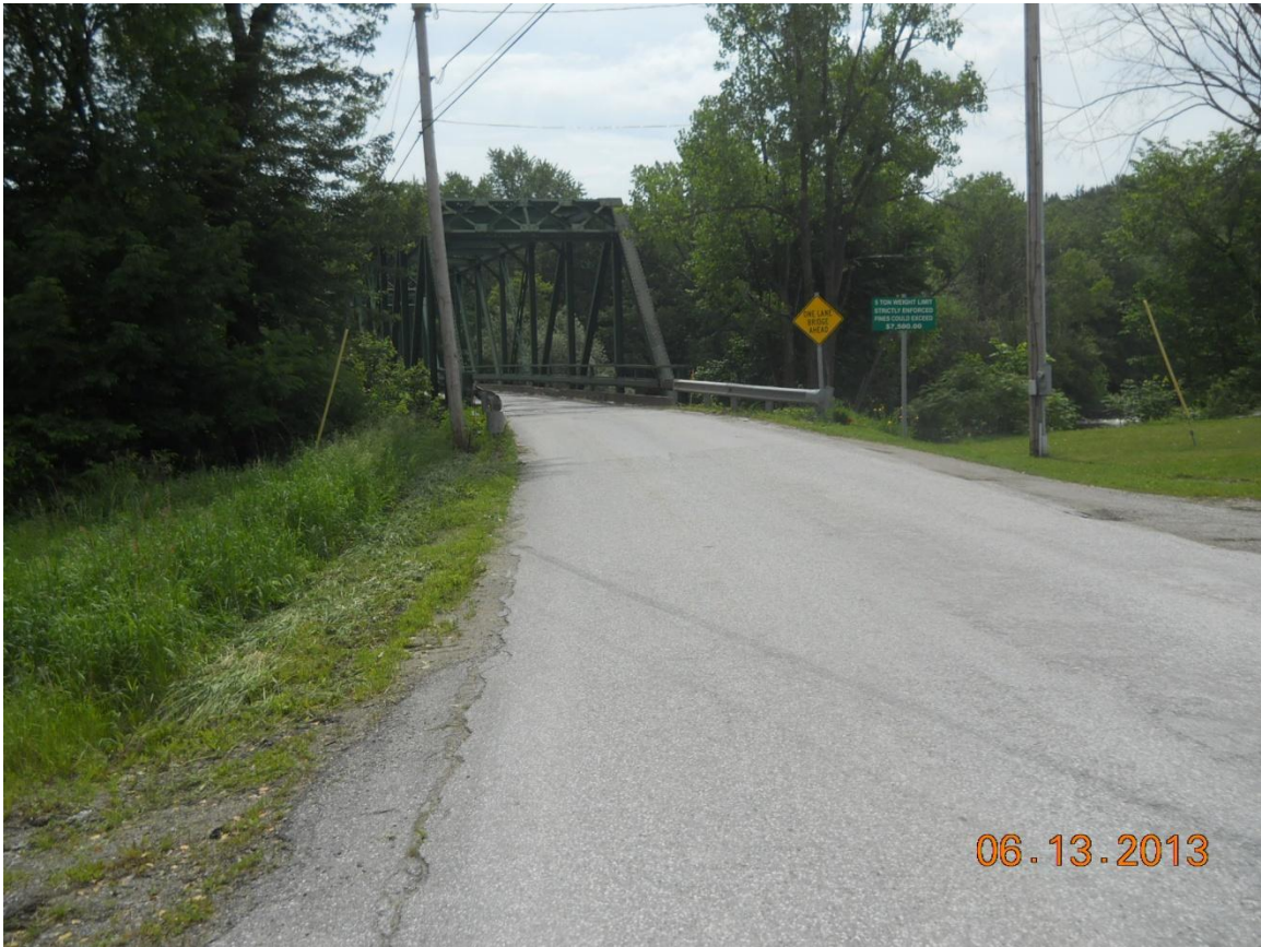
Looking East – showing narrow width and poor sight distance
