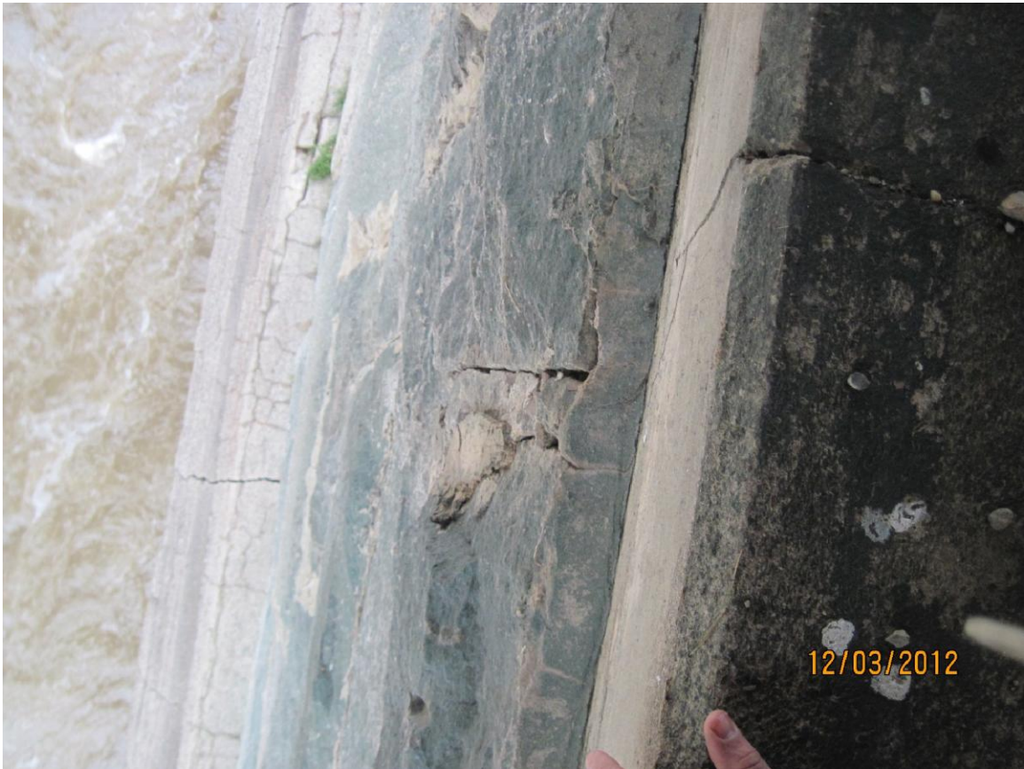
Additional Pier Cracks Continuing to form
