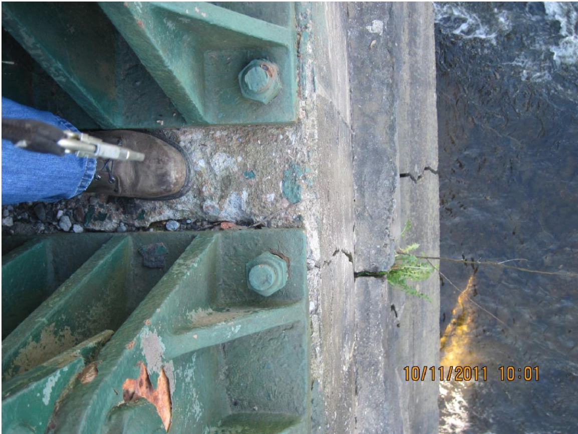
Pier Crack Before Patching
