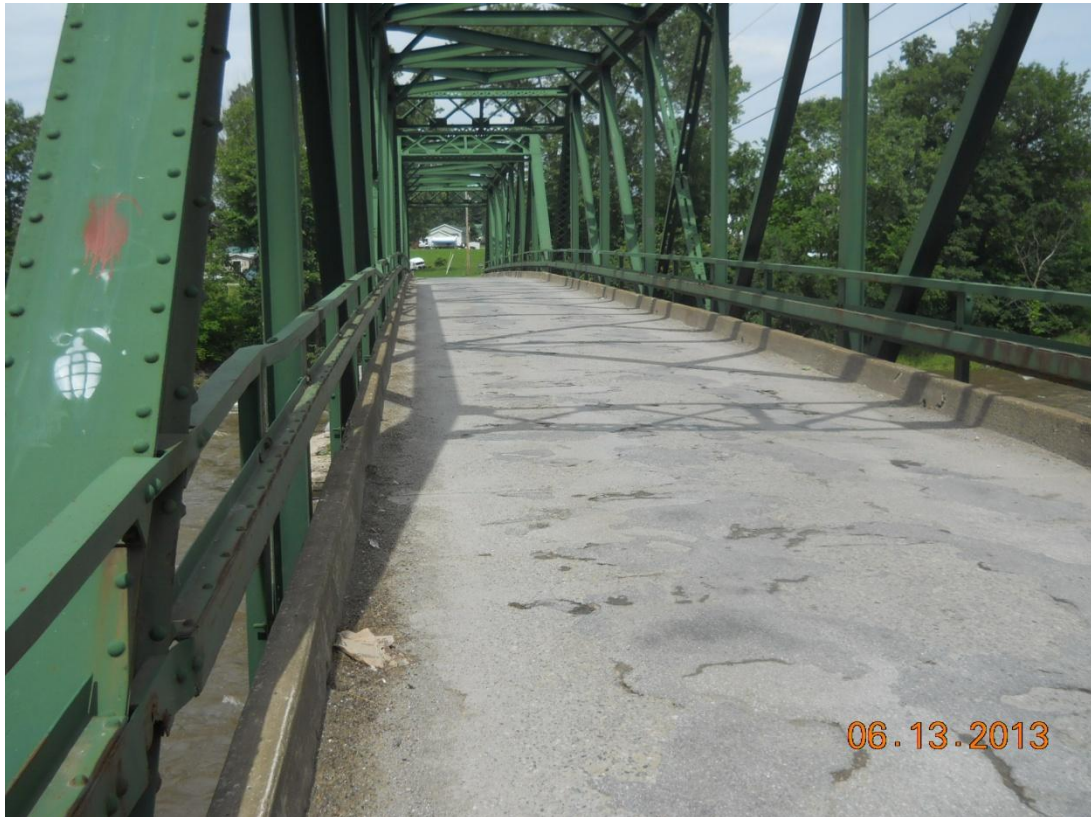
Looking West Across Bridge – Poor Condition of Deck and Pavement, Impact Damage, Narrow Bridge, Overhead Restrictions and Poor Sight Distance
