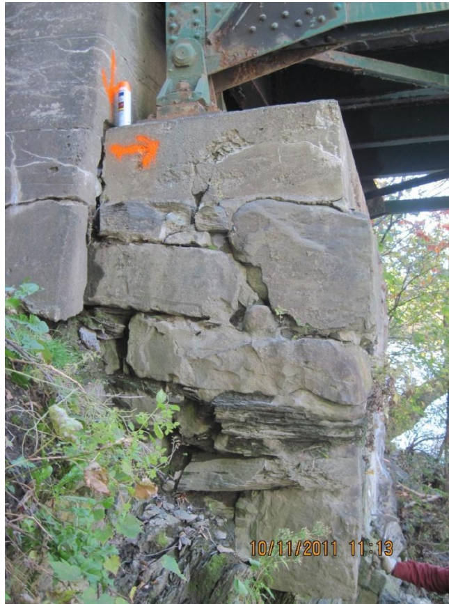
Eastern Abutment Slide and Settlement Failure
