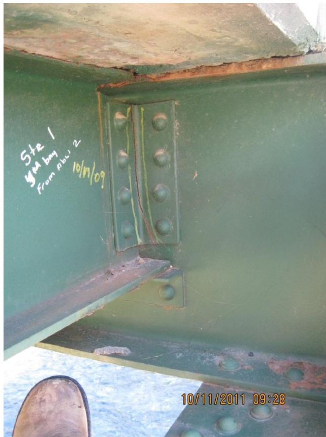
Cracked Stringer Connection Angle
