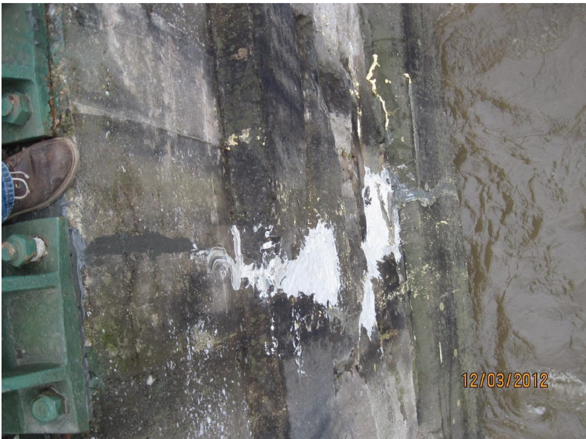
Pier Crack After Patching
