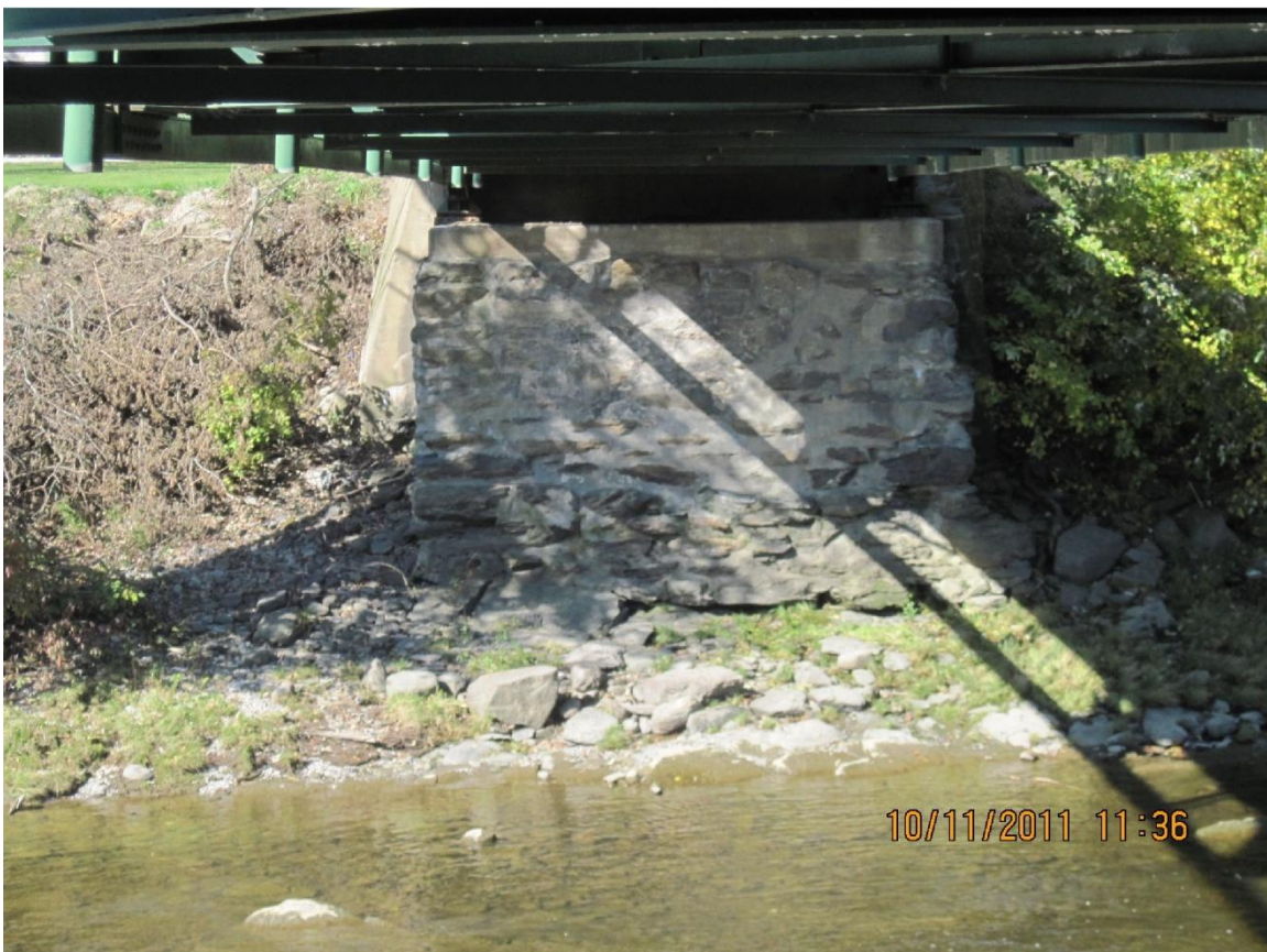
Western Abutment showing undermining
