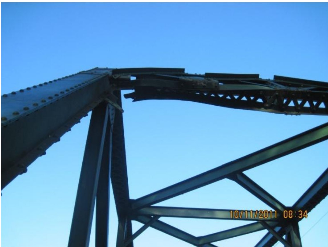
Example of Vehicle Impact Damage (End Portal Member)
